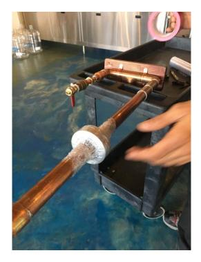
4. Both halves should be screwed to a full Disk without leaving a gap at any of both joints. If there is a gap, a device of bigger size has to be installed. Tighten the half's evenly and do not force the halves together by over tightening the screws. It is not necessary for the Pursanova Disk to fit exactly around the water pipe.
