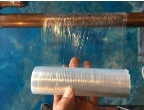
Pipe must be clean (free of any oils or residue)
