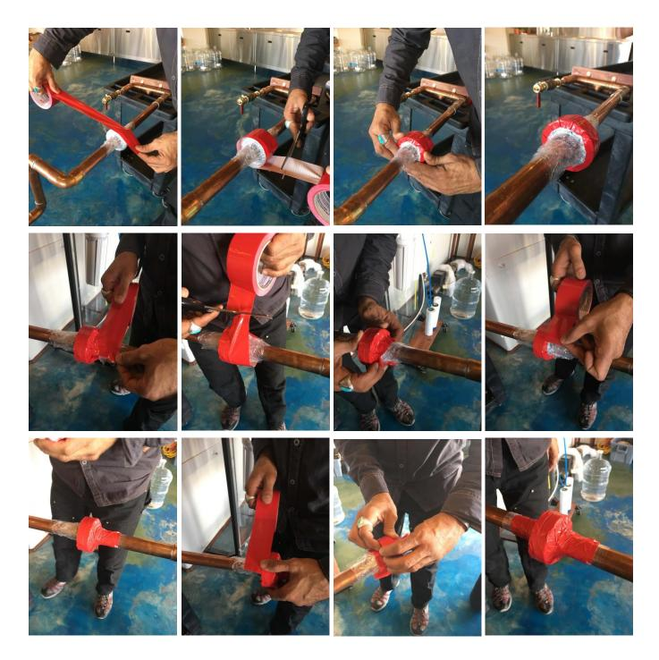
5. A gap between Disk and pipe does not impair the function of the Disk. When fitting the Pursanova Disk on the pipe, and the gap between the inside diameter of the Pursanova Disk, and the outside diameter of the pipe exceeds 5 mm, you must center the Pursanova Disk, on the pipe by using a non-metallic pipe wrap. Please avoid using any adhesive tape.
