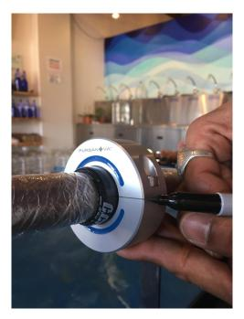
Close the gap evenly using the Allen Key and make it snug. Do not over tighten.
