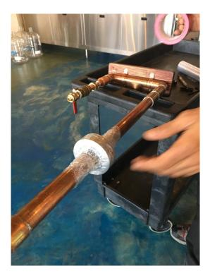
Press Plastic Wrap to make it fit tight around the Disk and the pipe.
