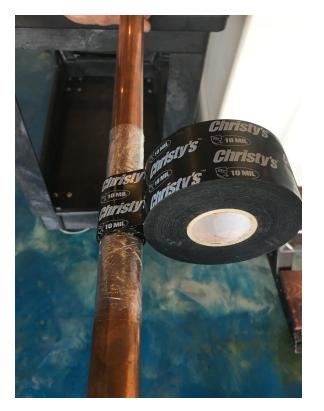
Wrap with Plumbers Tape to a thickness of about 1/4 inch.
