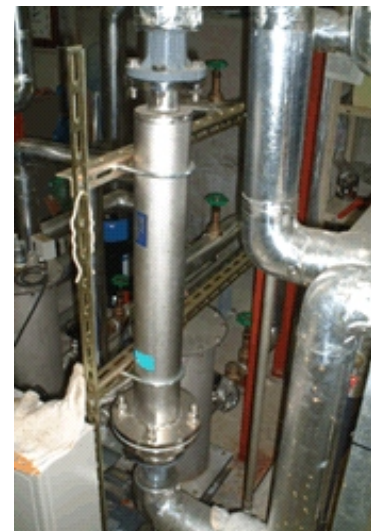
Installed C - 80 S
