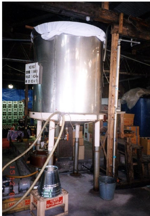
Installed at Condensation Control TS-1100 x 2
