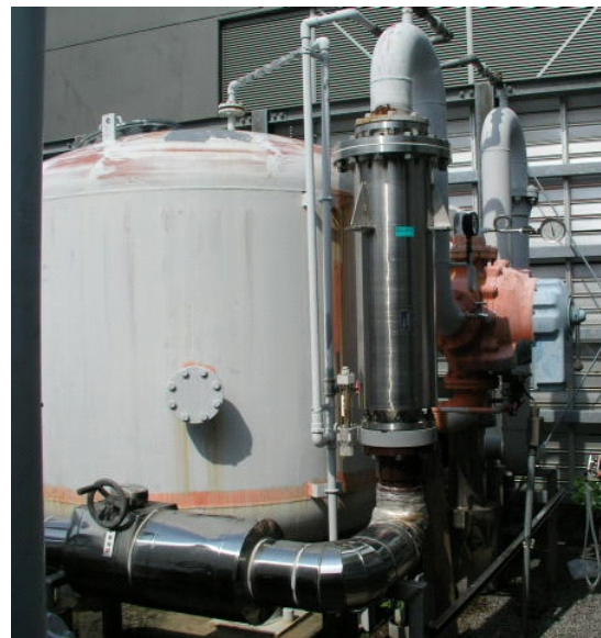
For 25m swimming pool Outdoor swimming pool (Filters 1 ton per minute) TC - 250S
